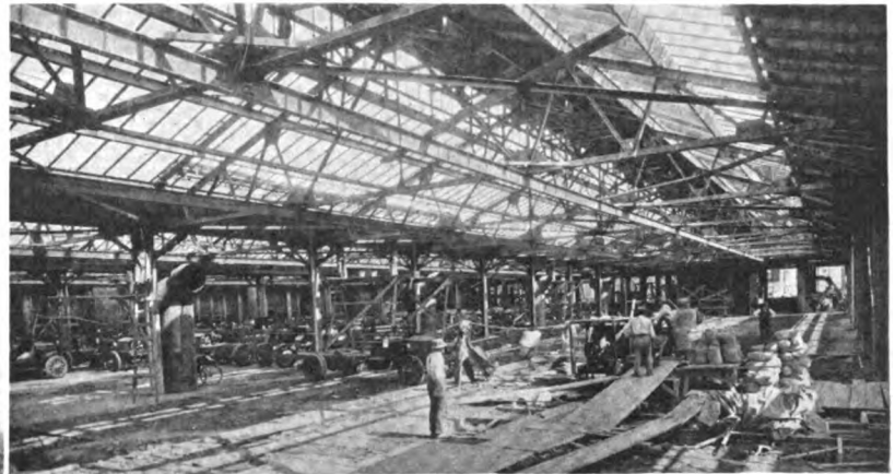
Above—Interior of the new truck erecting department of the Packard Motor Car Co., Detroit, Mich. This building is 240 ft. square and of steel and glass construction. As shown in the illustration, over 100 trucks were run in on the completed portion of the new floor and given final adjustment as fast as the cement dried
